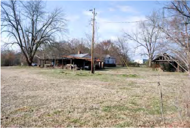
Photograph 044 Southwesterly View of Main House and Associated Outbuildings
