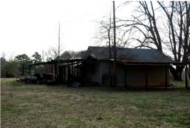
Photograph 007 Southwesterly View of Northeast Oblique
