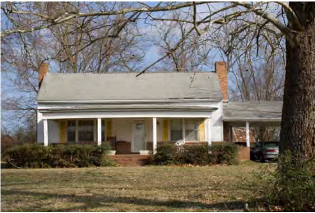
Photograph 001 Northerly View of Front (South) Façade
