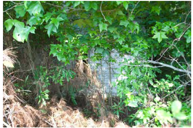
Photograph 028 Westerly View of Rear (East) Façade
