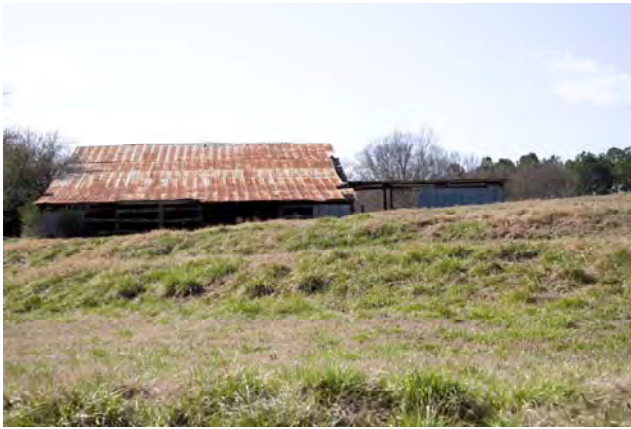
Photograph 025 Southwesterly View of Northeast Facade
