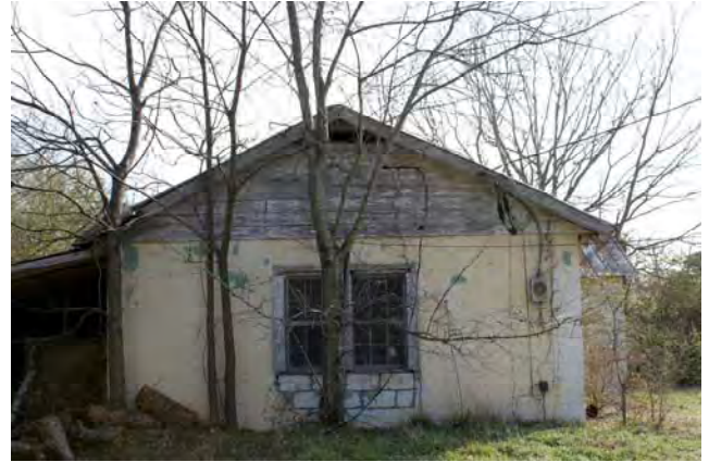
Photograph 012 Easterly View of West Facade
