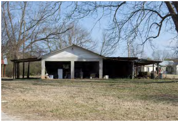
Photograph 6: Front (Southwest) Façade of Resource 2
