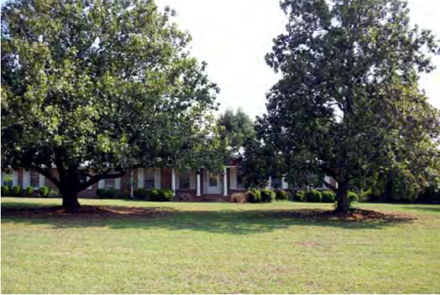
Photograph 035 Northerly View of Front (South) Facade
