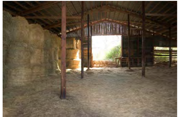
Photograph 10: Interior View of Resource 6
