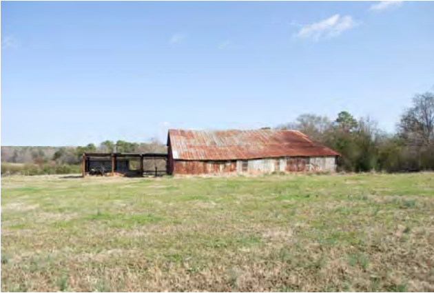
Photograph 020 Northwesterly View of Southeast Facade
