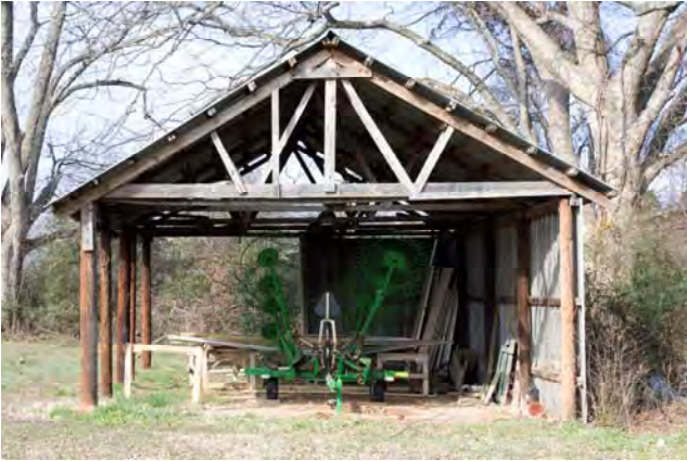
Photograph 008 Westerly View of East Facade
