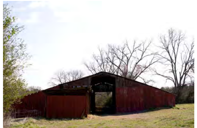
Photograph 023 Northeasterly View of Southwest Facade
