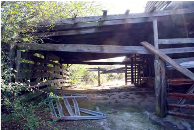
Photograph 017 Interior View of Mule Barn
