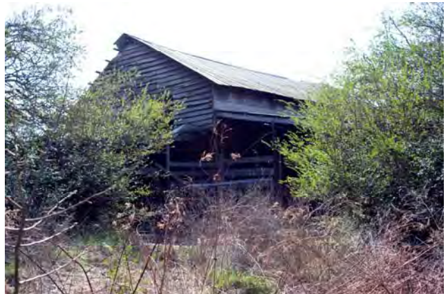
Photograph 018 Southeasterly View of Northwest Facade
