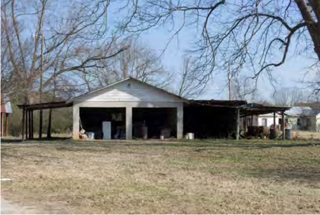
Photograph 005 Northerly View of Southeast Facade
