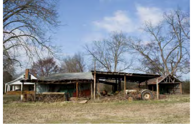
Photograph 006 Northwesterly View of East Facade
