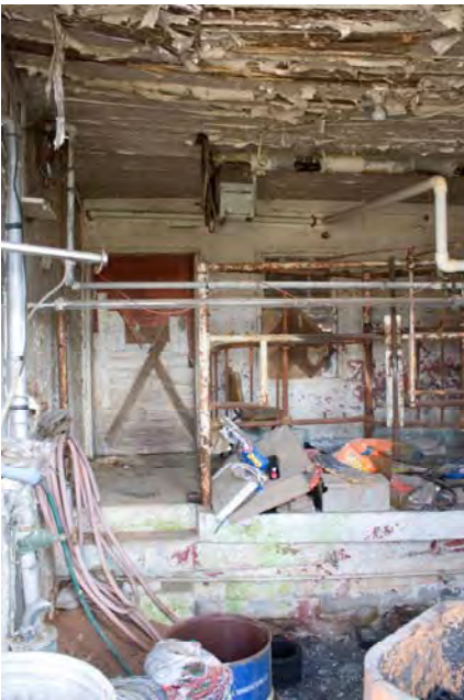
Photograph 013 Interior View of Milk House
