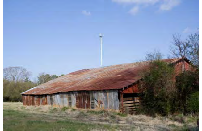
Photograph 021 Southwesterly View of Northeast Oblique
