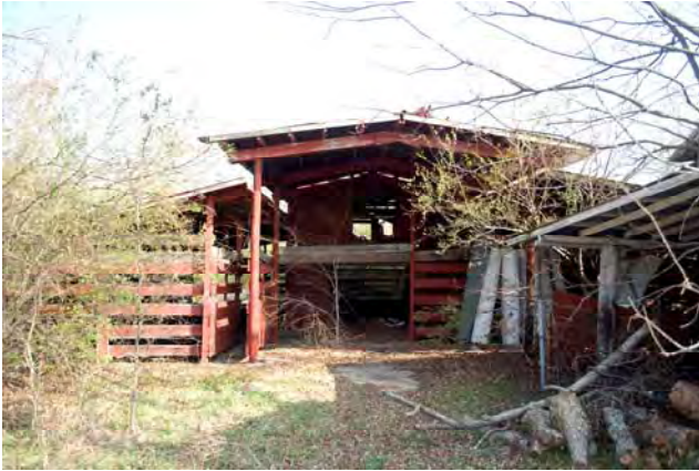
Photograph 015 Northeasterly View of Southwest Facade
