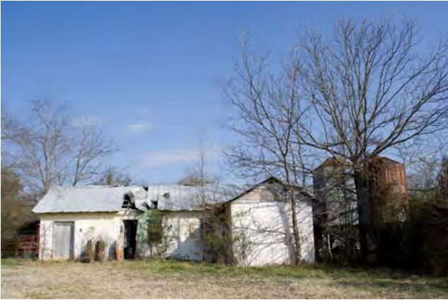
Photograph 011 Northerly View of Front (South) Façade and Silos
