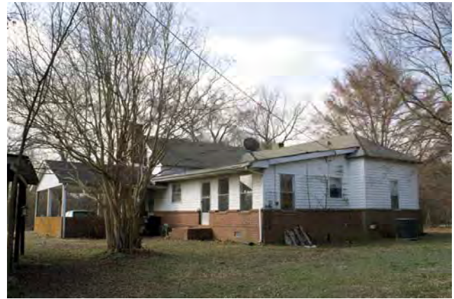
Photograph 004 Southwesterly View of Northeast Oblique
