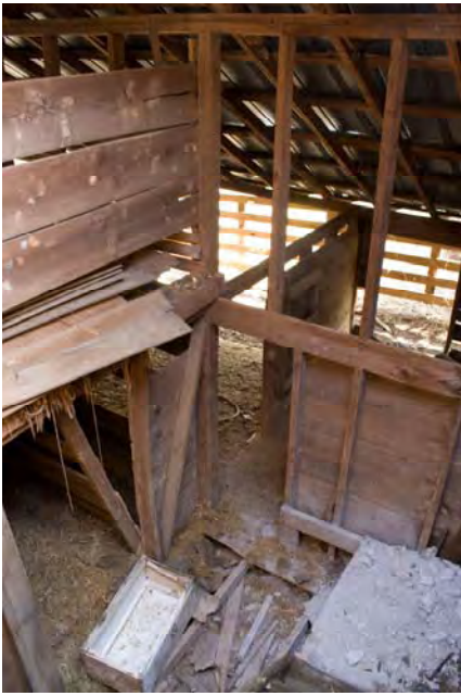
Photograph 019 Interior View of Mule Barn
