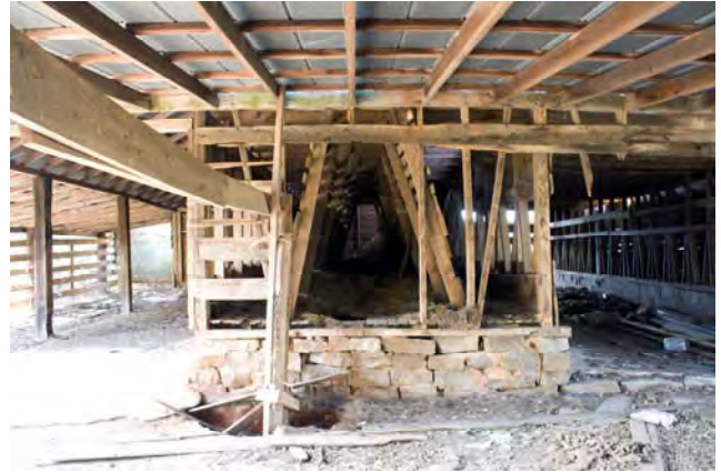
Photograph 016 Interior View of Mule Barn
